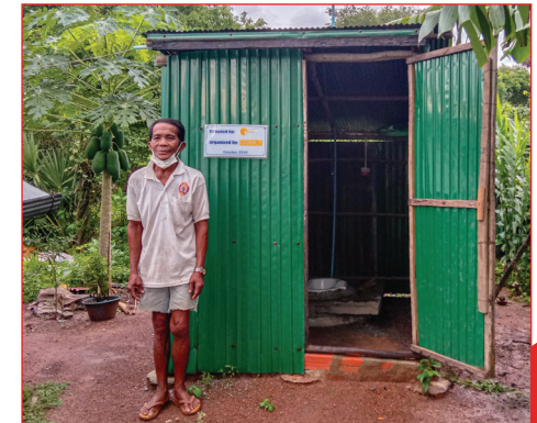
Toilet building for Pich Nheob and her husband.
